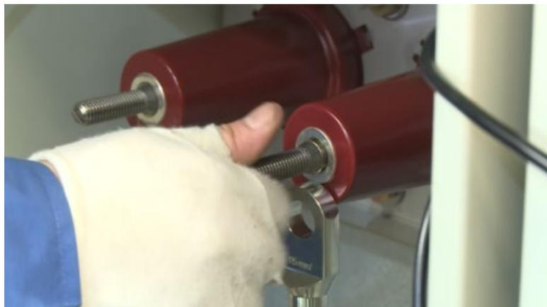
Figure 3- 18 Insert lugs onto each phase conductor
