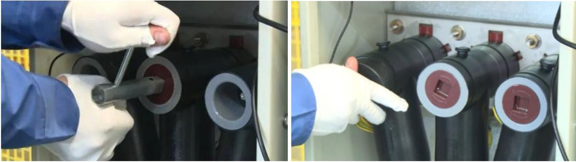
Figure 3- 22 Install the nut and washer
