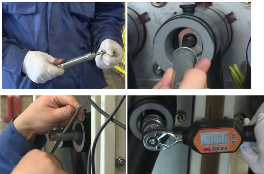
Figure 3- 21 Push Tee connector and cable adapter into bushing
