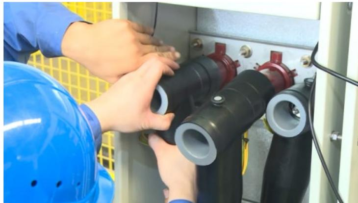
Figure 3- 20 Push cable into Tee connector
