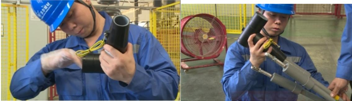
Figure 3- 19 Clean and apply grease
