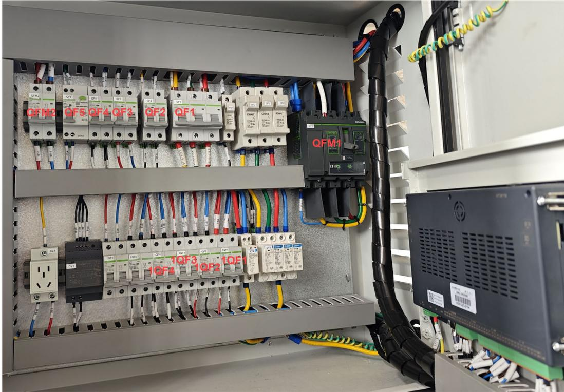
Figure 4- 3 Circuit breaker of battery container
